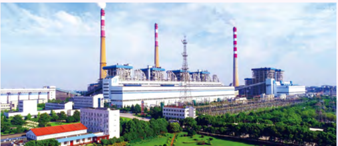
Huaneng Yangluo Power Plant
