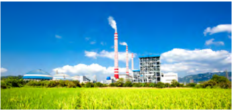
Fuzhou Power Plant
