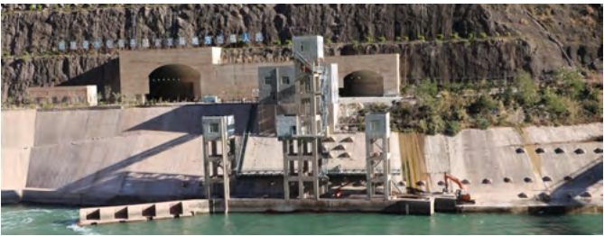
Fish Lifting Facility at Huangdeng Hydropower Station
