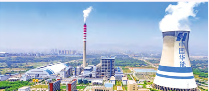
Huaneng Jingmen Thermal Power Plant
