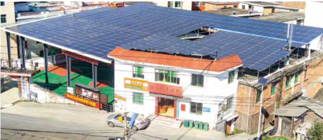
185kW PV Power Project in Huhe Village, Longyan City
