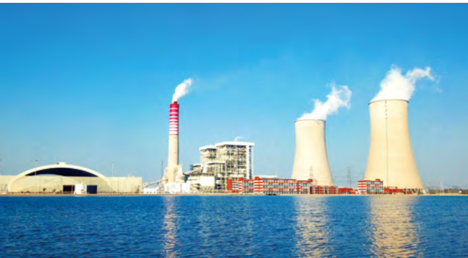
Huaneng Sahiwal Coal-fired Power Plant
