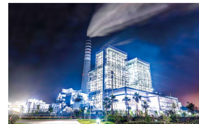
Luoyuan Power Plant
