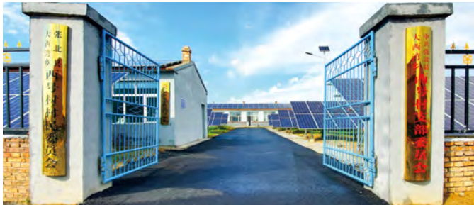
Distributed PV Power Project in Xihao Village, Zhangbei County
