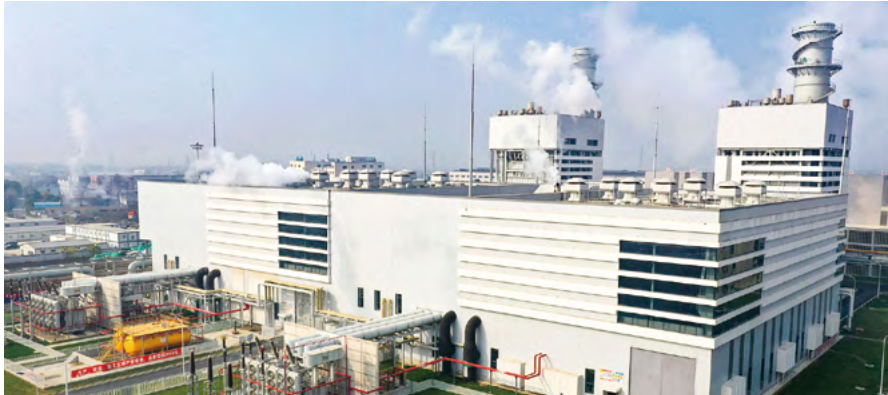
Jiangyin Gas Turbine Thermal Power Co., Ltd.
