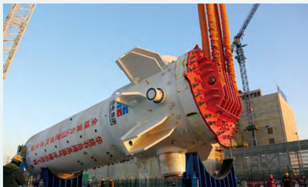
The First Steam Generator was Lifted into Place
