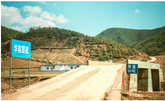
Safety Bridge in Tuanjie Village, Zhaojue County
