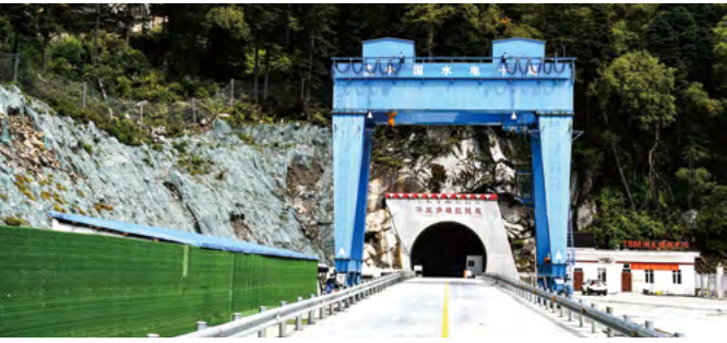
Entrance of the Duoxiongla Tunnel
