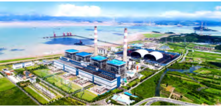
Yuhuan Power Plant
