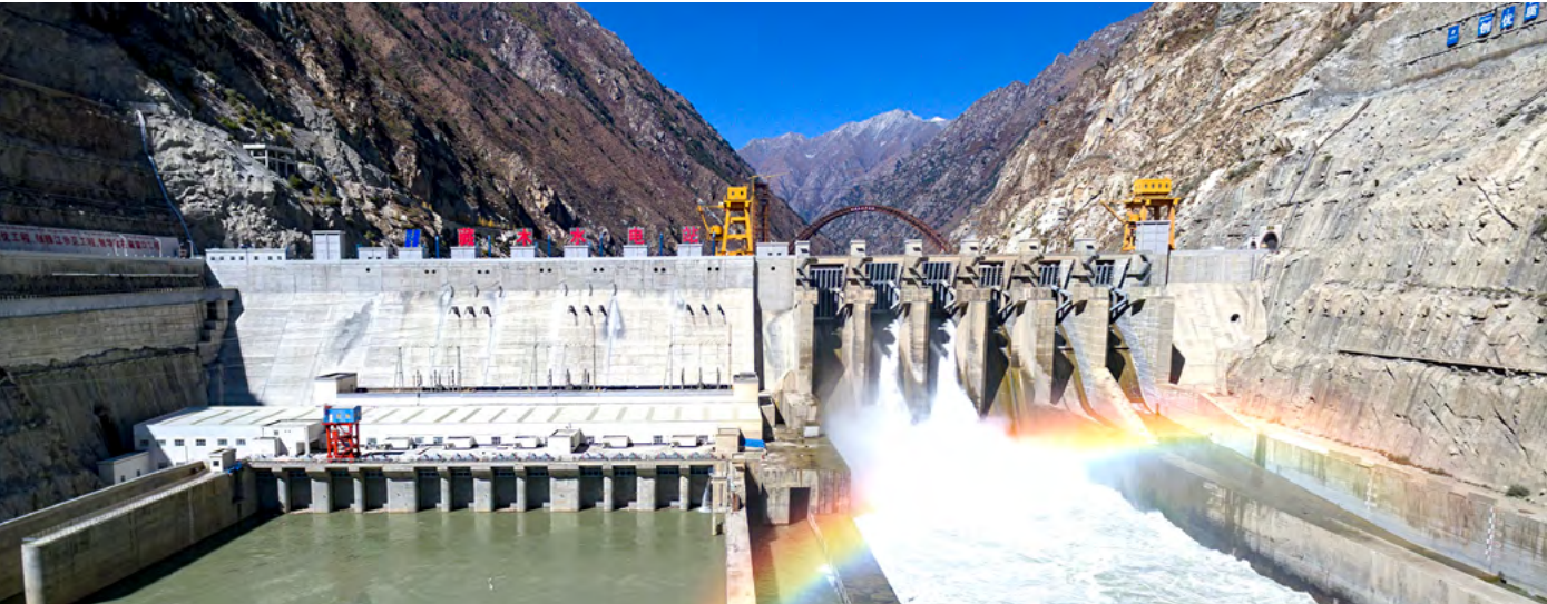
Zangmu Hydropower Station
