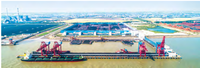
Huaneng Coal Terminal Project - Taicang Port Area, Suzhou Port
