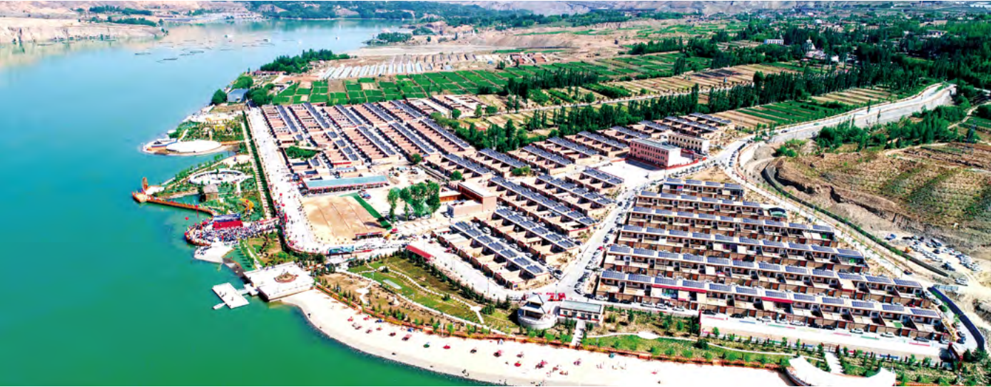
Roof Distributed Photovoltaic Power Project at Relocation Site in Dej Village
