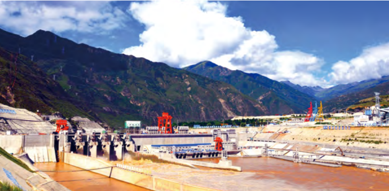
Gyaca Hydropower Station
