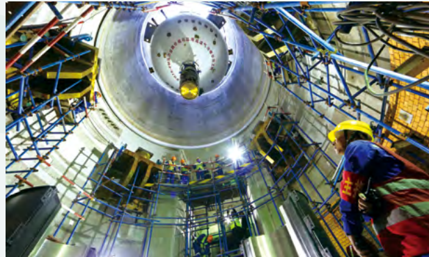
The First Reactor Pressure Vessel was Lifted into Place
