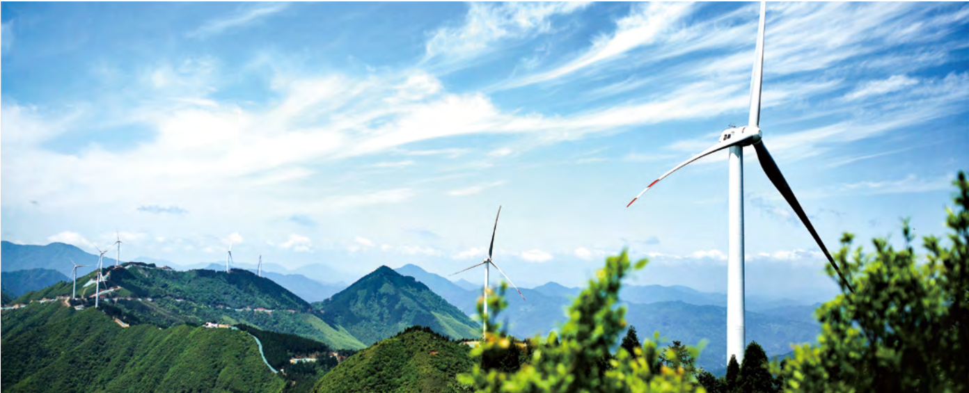
Gaolong Hill Wind Farm
