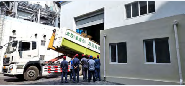
Sludge Power Generation Project of Qinre Power Generation Co Ltd.
