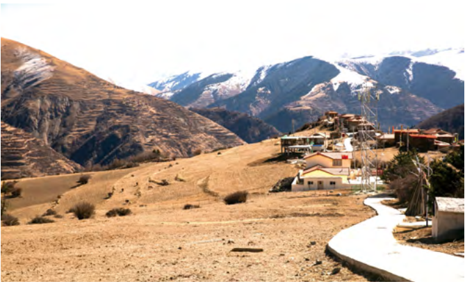
Household Hardening Road in Yanggao Village, Aba County
