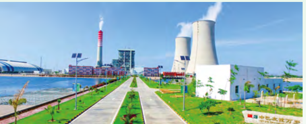
Green Huaneng Sahiwal Coal-fired Power Plant
