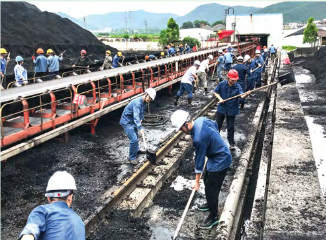
Cleaning and Strengthening of Coal Yard in Huaneng Jinggangshan Power Plant
