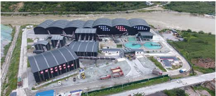
Aggregate Processing Area of Yingliangbao Hydropower Station
