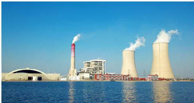
Huaneng Sahiwal Coal-fired Power Plant
